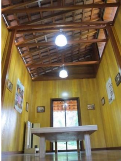
Figure 2. Interior of the CLT structure
