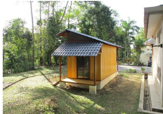
Figure 1. Front and rear elevation of the CLT structure
