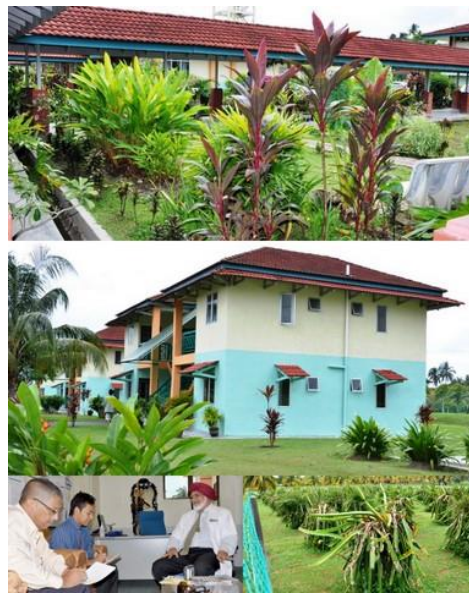
Figure 6.2 Surrounding Views of Hospital Bahagia, Ulu Kinta, Perak (Source: Image by HBUK)
