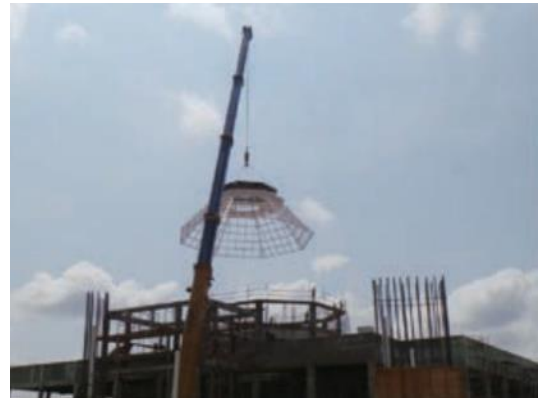
Figure 7: Placement of the dome structure using a mobile crane
