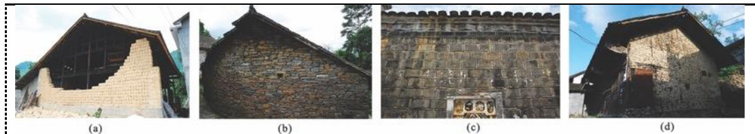
Fig. 9. Materials of building (a) earth (b) stone (c) brick (d) bamboo walls with cattle dung and mud
