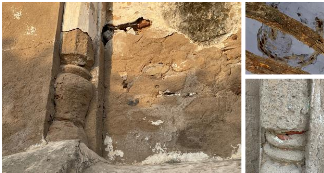
Fig. 8. Different building materials of the mosque: Lakhori bricks, stone rubble masonry, and lime mortar (Source: Nitya Bali)
