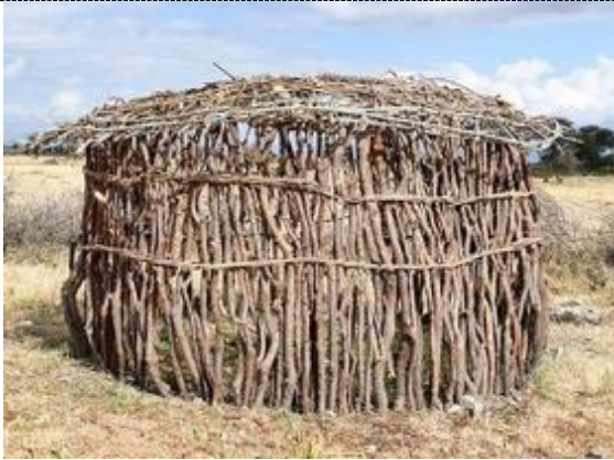
Fig. 6: The structure of a traditional Manyatta made from sticks
