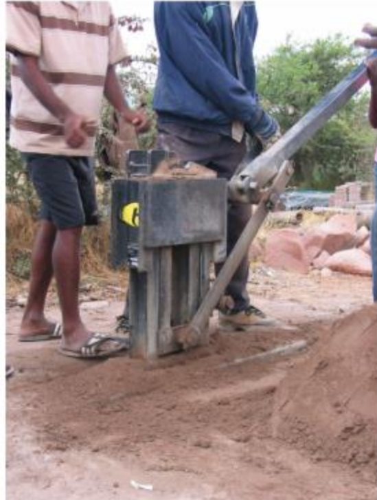
Fig. 31. Construction of compressed earth blocks (CED) using a hand press
