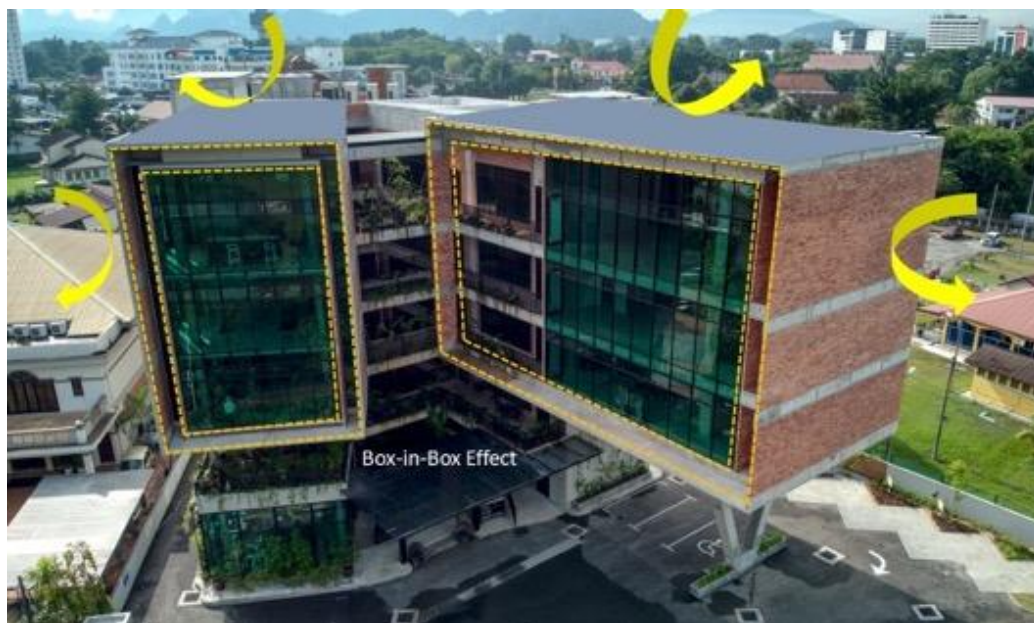
Fig. 23. The box-in-a-box effect prevented heat from the east and west from penetrating into the building. When combined with the thick roof insulation, temperatures within the building was kept highly stable.
