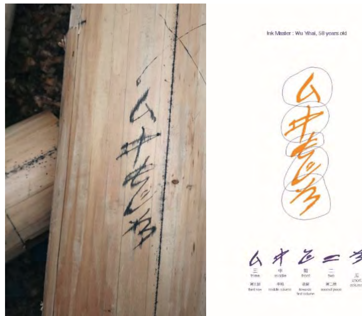
Fig. 5. Set of characters and symbols on timber components
