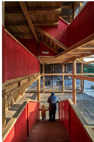
Fig. 11. Insertion of main staircase within traditional Dong house framework
