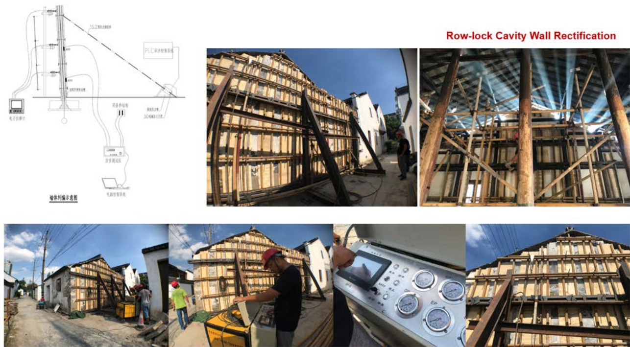
Fig. 13. Row-lock Cavity Wall Rectification based on the principle of minimal intervention
