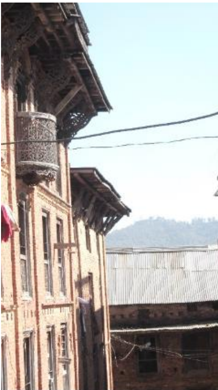
Fig. 21. (Pic Source: Sakar Shrestha) A rare Cantilevered curved wooden balcony with carved railing
