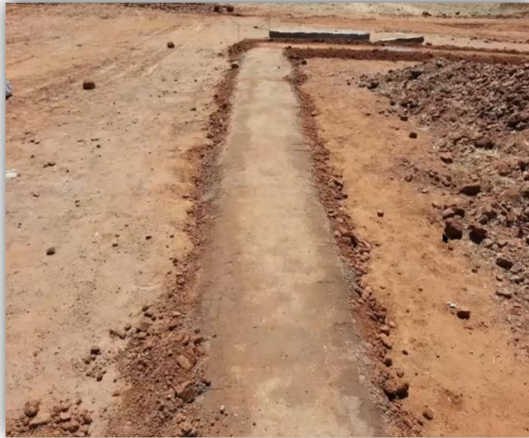
Fig. 7. Stabilized Rammed Earth Foundation used in Building Construction of Dhamma Arunachala. Source: (Gopalan, 2022)
