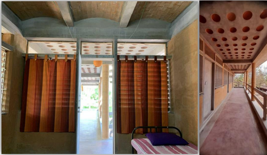
Fig. 9. Jack Arch Vault (Left) used as a floor system in the room and Filler Slab (Right) used in floor slab system in the corridor. Source: Author
