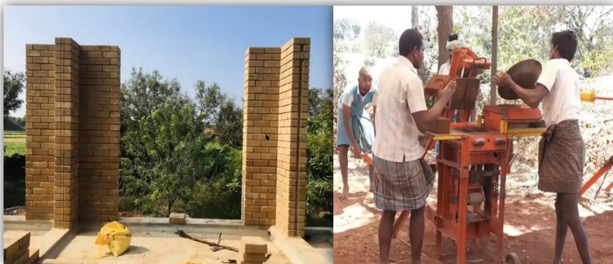
Fig. 8. Compressed Stabilized Earth Blocks (Walls) and Auram-3000 used to produce CSEB Source: (Gopalan, 2022)
