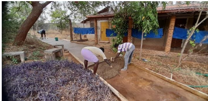
Fig. 24. The pathway paved with Earthen Concrete. Source: (Gopalan, 2022)
