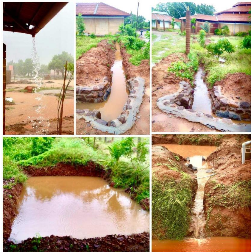
Fig. 23. Ground Water Recharge by the Rain Water Harvesting through the pond. Source: (Gopalan, 2022)
