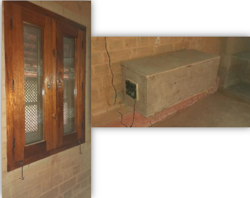
Fig. 17. Double Glazed Windows in the main Meditation Hall (Left) and Lower Powered Fan for forced ventilation (Right). Source: Author
