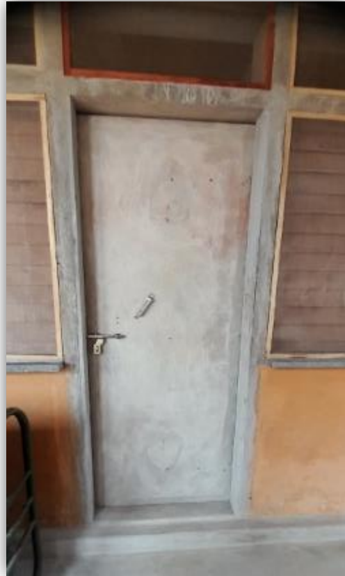
Fig. 11. Door using Ferrocement shutter. Source: Author
